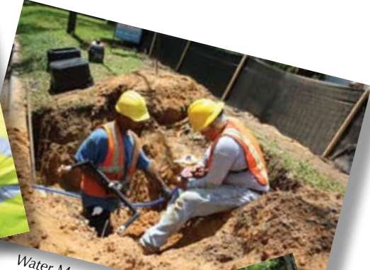
Water Meter Repair
