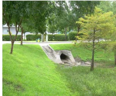
**Grassed swales** can be found directing storm water around buildings and towards the pond. Inlets are found in parking areas, depressed green spaces, and curbs, and are usually underground conveyances directing the runoff into the pond.
